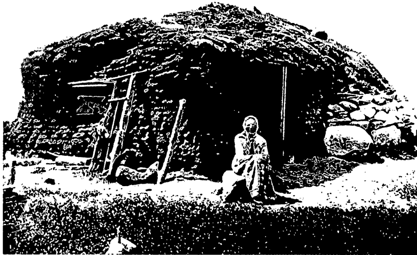
Sod houses, like this one built in the 1870s by Norwegian settlers near Madison in Lac qui Parle County, were warm in winter and cool in summer. Since few trees grew on the prairies of western Minnesota, the pioneers there built houses and sheds by cutting the thick sod into rectangular pieces and laying them like large bricks. Sometimes sod huts were built half underground or dug into the side of a hill for protection against the winter blizzards. (Courtesy of Lac qui Parle County Historical Society)
